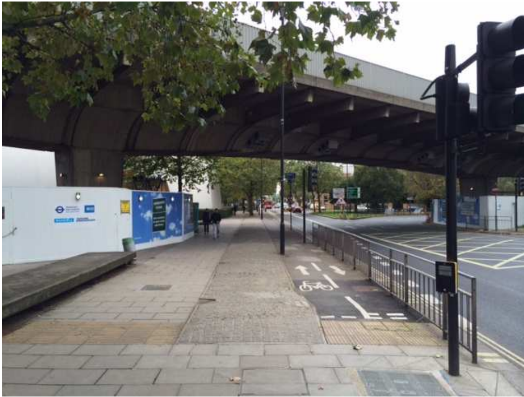
Photo 1 - Existing segregated cycle lane to be widened
